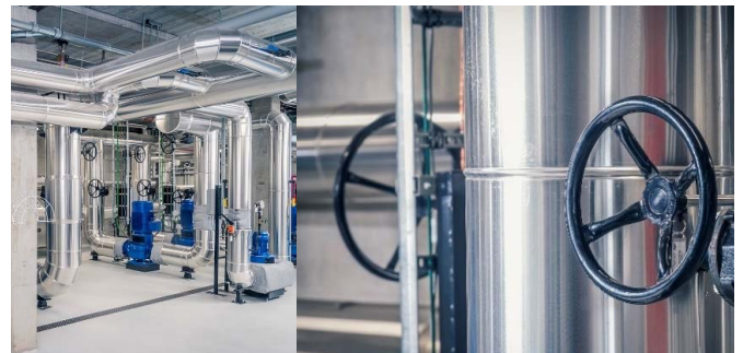
BROEN Ballomax® ball valves controlling the flow of district heating water
