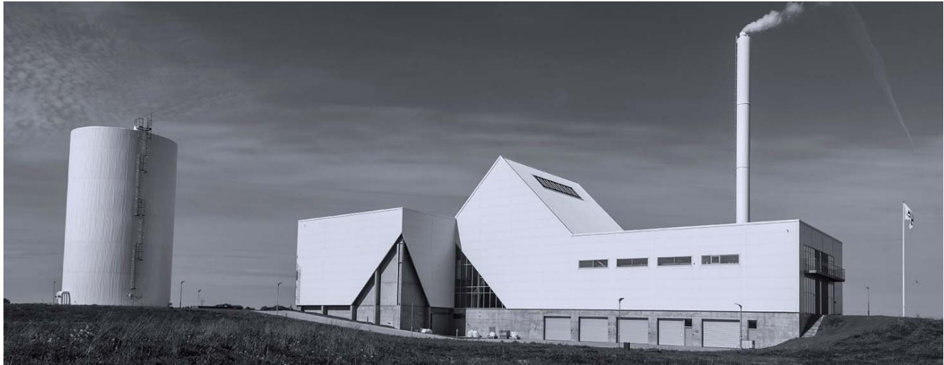
Aabybro district heating plant (Denmark).
